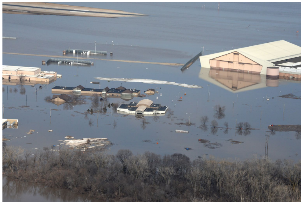
Water covers one-third of Offutt Air Force Base, Nebraska, after the Missouri River flooded in March 2019.
