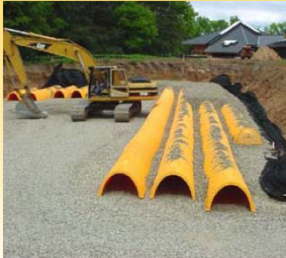
Minnesota Stormwater Manual
